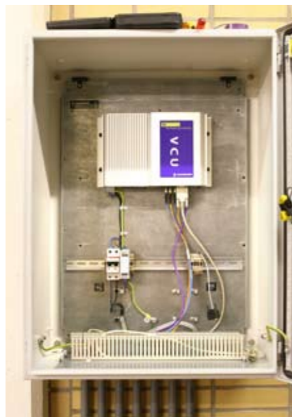
The VCU box is placed in a wall mounted sheet steel cabinet with one front door. All cabling, such as power supply cable, fiber optic cables and data communication cables are fed into the cabinet from the bottom.
