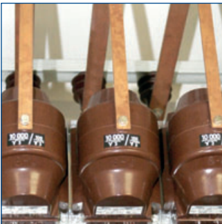
The SASensor Voltage Interface Module can be connected to all conventional voltage transformers.
